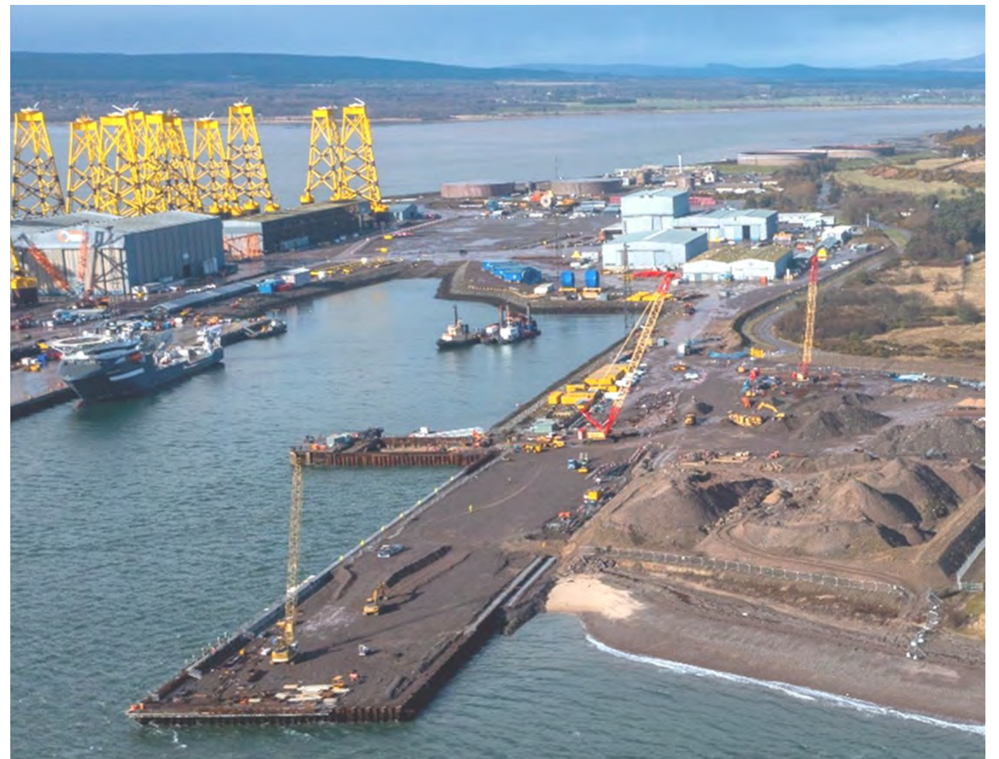
Elevated view from the south east
