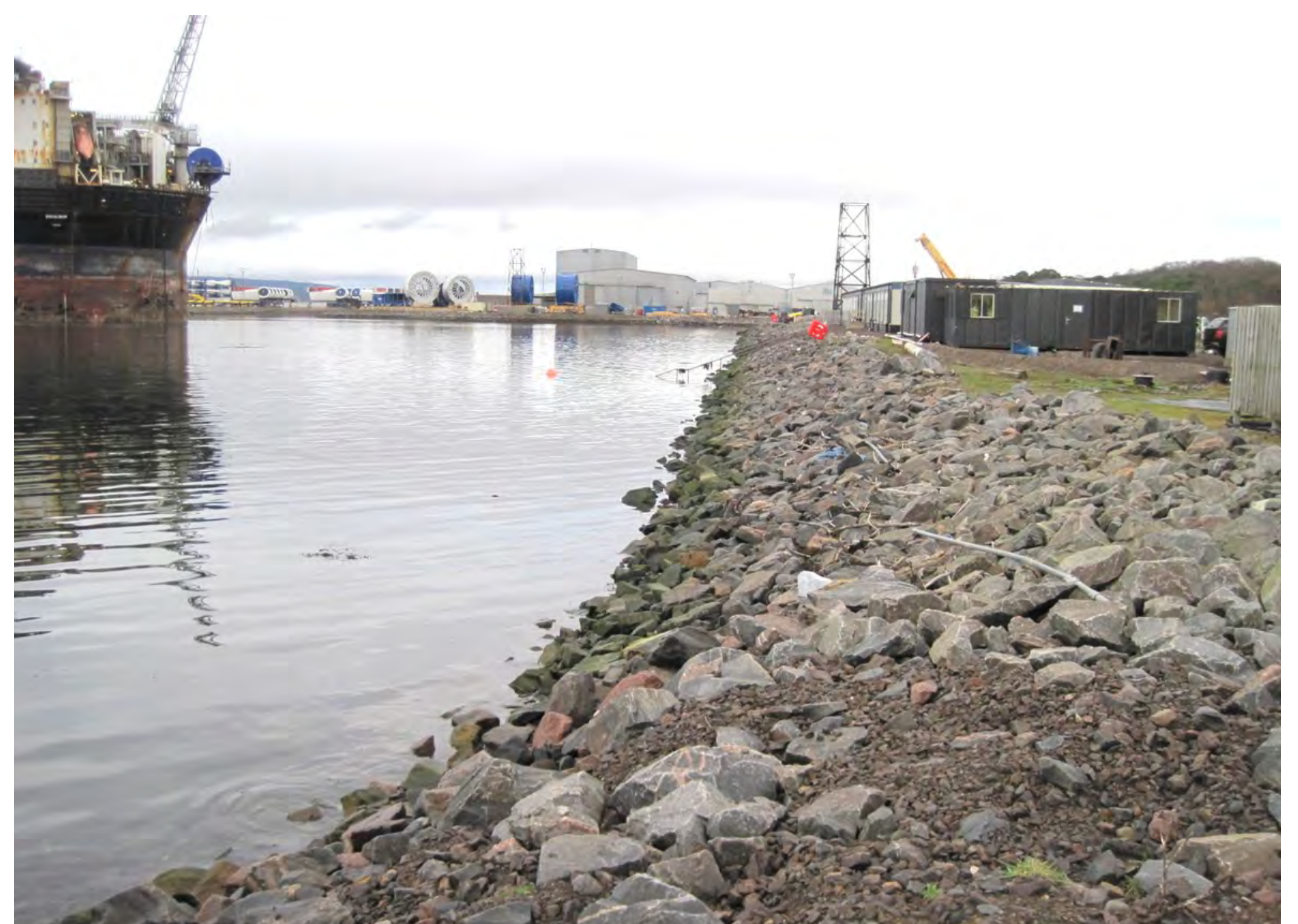
Current view from the south end of the Inner Dock
